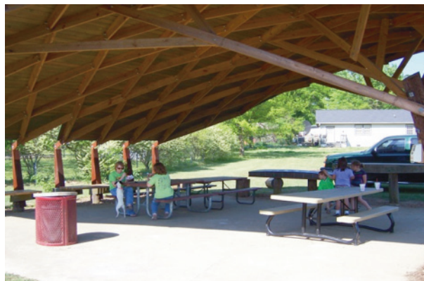
Figure 2. Recreational facilities utilizing preservative-treated wood. Top, a ramp for scaling a bluff at a state park. Bottom, a city park pavilion.
