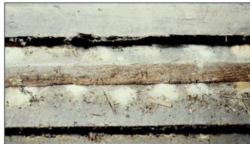
Figure 6. Powderpost beetle frass may accumulate in piles beneath exit holes.
